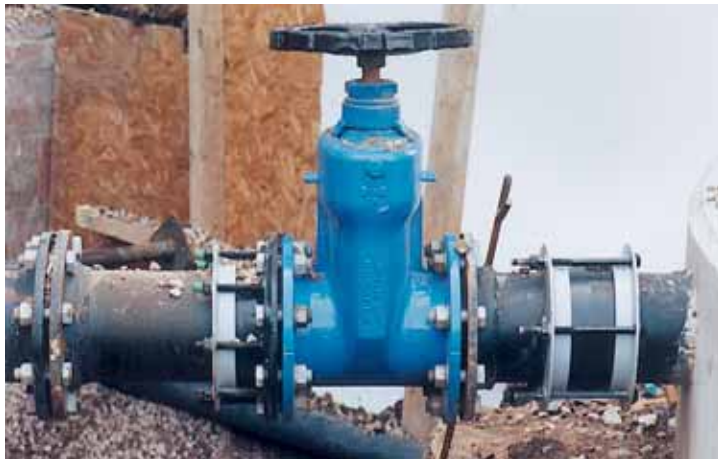
170mm FlexLock coupling and flange adaptor used to install a valve.
